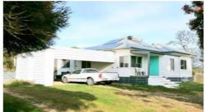
HOUSE & CARPORT, SOLAR PANELS
