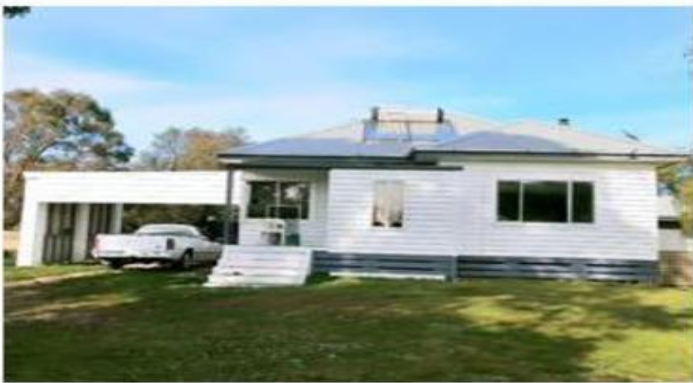
FRONT OF THE HOUSE & SOLAR HOT WATER
